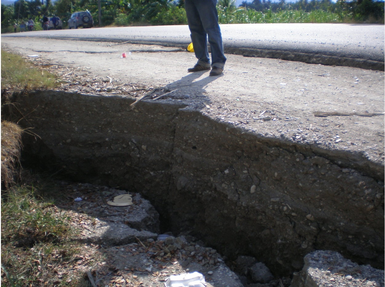
Figure 8.6 Well-compacted granular fill at road damage site BOXCLVTA.
